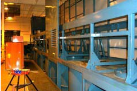
Photo 1 looking down the line
